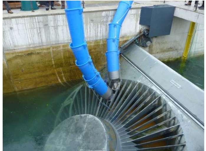
Position at the median point (mid-blade) on the left and external (at the runner periphery) on the right
