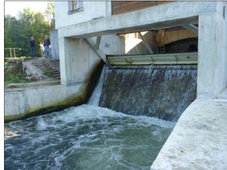
Downstream view of the Frouard HPP tailrace
