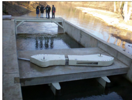
Saint Jean de Rives after renovation
