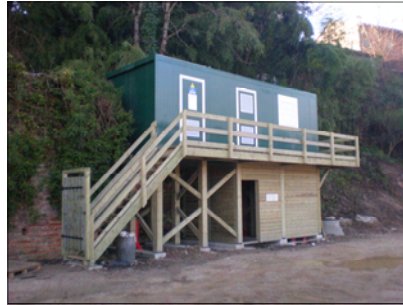
St Jean de Rives equipment room
