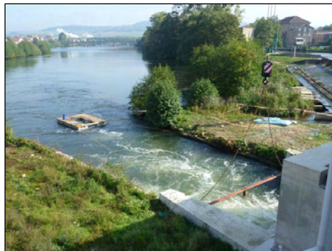
Installation of the recovery device: net frame, net, and floating pontoon
