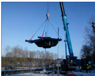
Installation of the Ame VLH in January 2010
