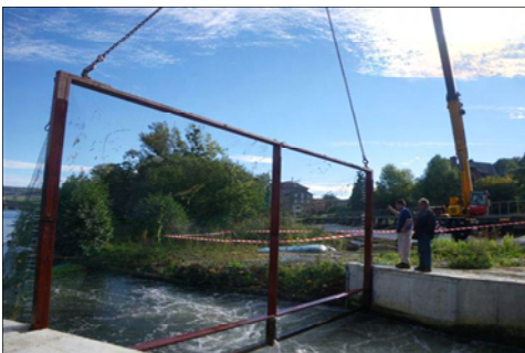
Installation of the net by means of the crane
