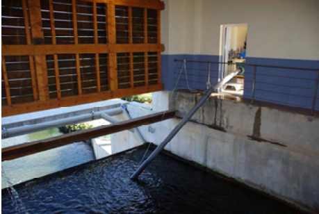
VLH in operation, with installed injection system
