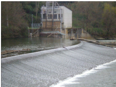
Saint Jean de Rives before renovation
