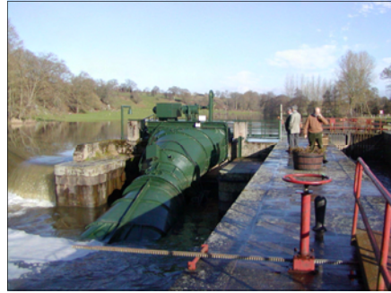
Typical existing Mayenne plant
