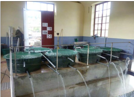
Storage tanks with weirs
