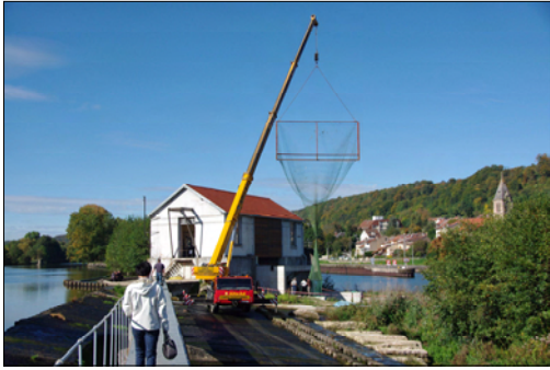
General view of the Frouard SHP
