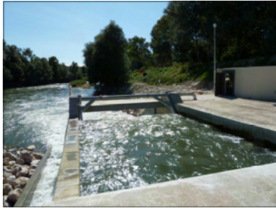
Montodine power plant, South of Milan A VLH DN 4500 and 500 kW
