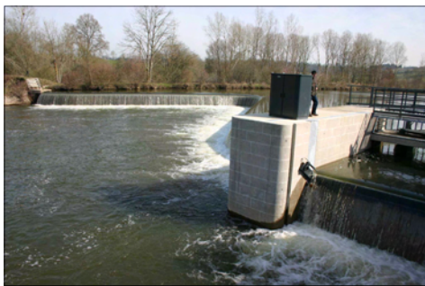
L'Ame SHP downstream view
