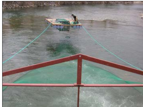
Installation of the recovery platform and of the net
