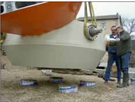
Runner craned on assembly area
