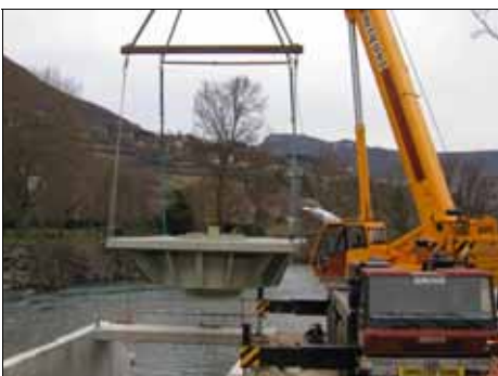
Horizontal rotation towards the VLH location
