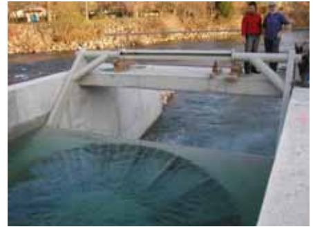
The VLH in operation connected to the grid
