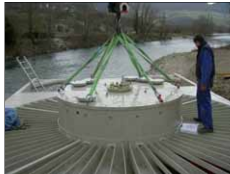
Assembly of the generator inside the distributor on top of the runner
