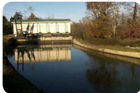
Barcelone de Gers plant before the starting of erection
