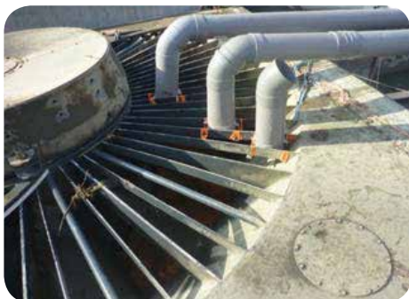
Injection device on the VLH DN 5000 in Yennes
