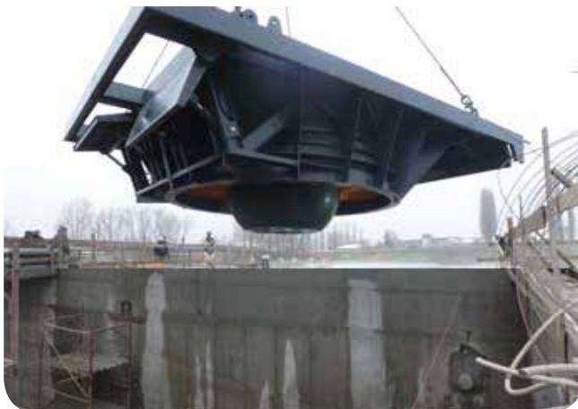
One of the 2 VLH DN 5000 in Isola Dovarese
