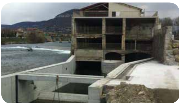
Delivery of La Glacière HPP in Millau (France)
