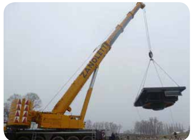
Lifting of a VLH on its final position
