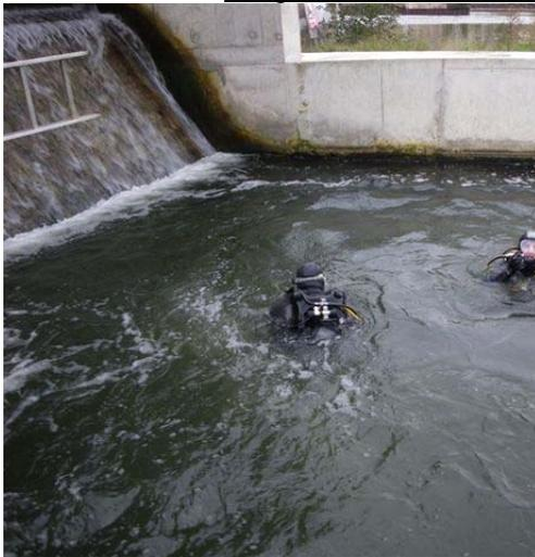
Image 9. Divers inspecting the junctions between the concrete parts and the frame
