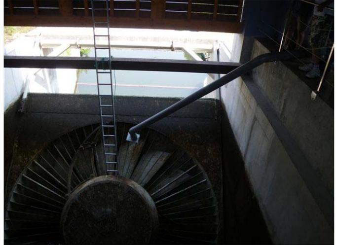
Image 4. View of the injection tube connected to the metal part installed on the VLH distributor , the turbine chamber being empty
