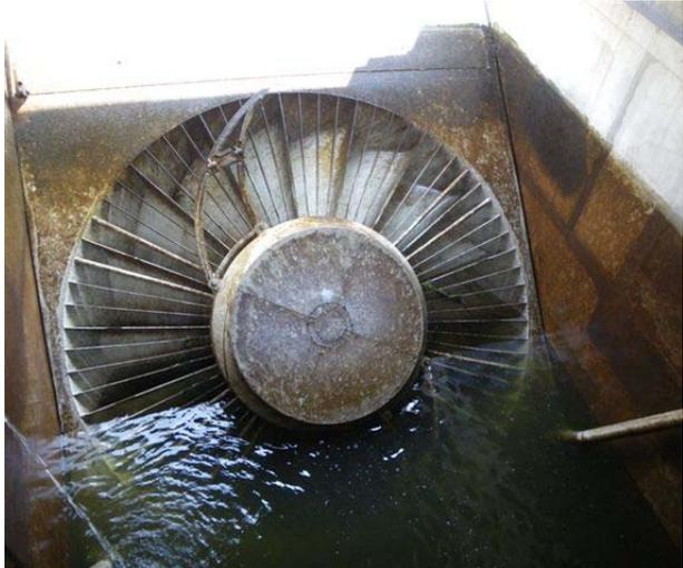
Image 1. The lock power plant VLH in Frouard as the turbine chamber is being emptied
