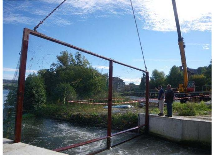
Image 16. Installation of the frame by means of the crane
