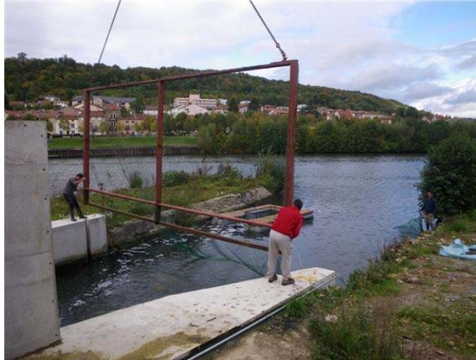
Images 7 and 8. Frame supporting the net installed with the crane
