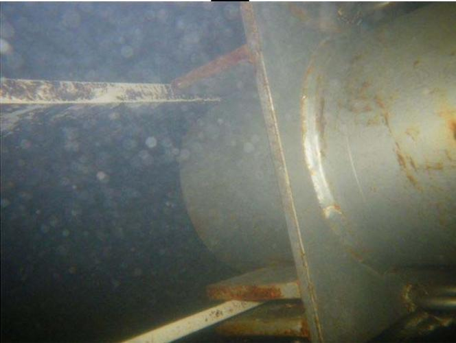
Image 5. Underwater view of the installed metal part, astride the metal spokes of the distributor
