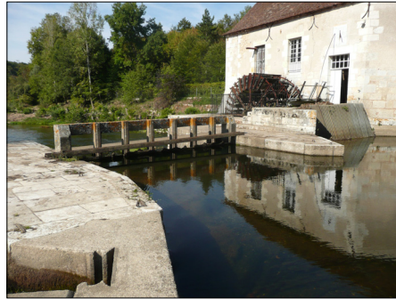
Bay where the DN 3150 VLH of the Fontgombault Abbey will be installed
