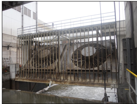
Upstream view of the structure in lifted position
