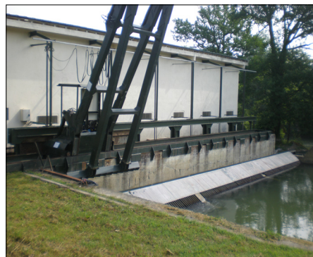
Upstream view of the Barcelone de Gers HPP
