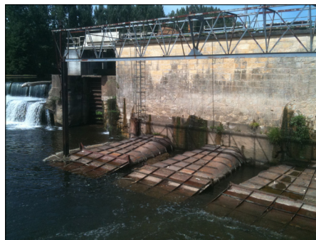
Downstream view of the Aubas HPP
