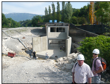
Civil Works of Yenne HPP
