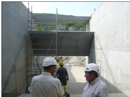
Concrete structure of the Yenne DN 5000 VLH
