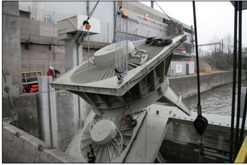
Craning of the 2 nd VLH in the supporting structure
