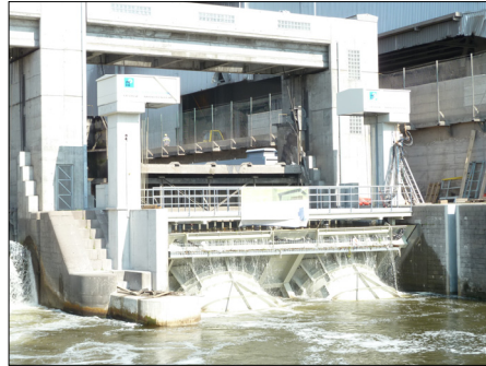
Downstream view of the VLHs and their supporting structure
