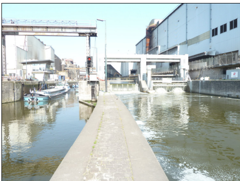
Downstream view of the VLH in operating conditions
