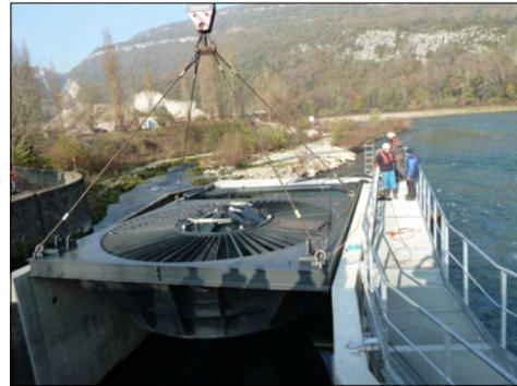
End of craning of the turbine into its concrete position
