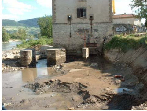
The working site is out of water The excavations can start
