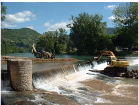
The downstream and upstream cofferdams almost join
