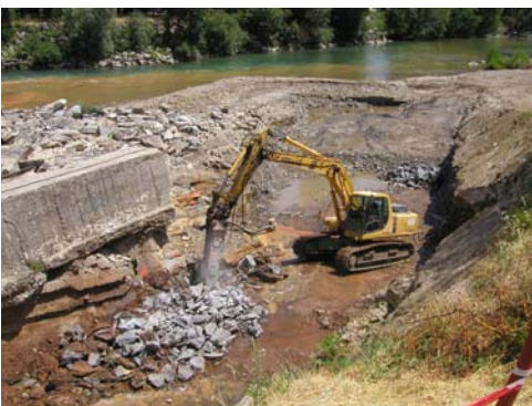
Downstream excavation at the VLH implantation level
