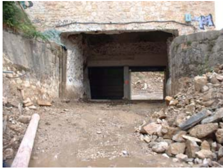
Completely clear water passage under the old building
