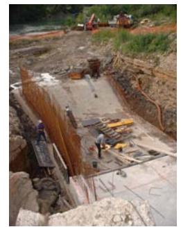
Lateral reinforcements at the level of the VLH unit
