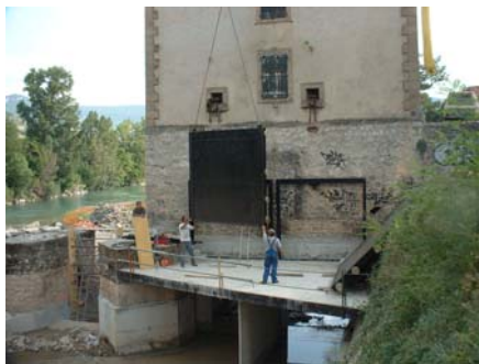
Installation of the frames of the upstream valves
