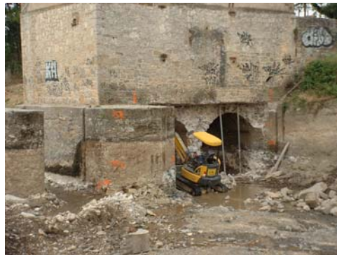
The excavations are over, below-grade demolitions start upstream
