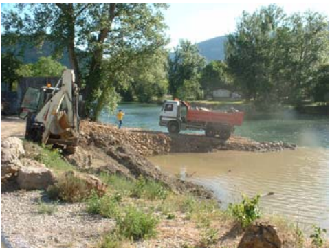
Construction of the upstream cofferdam
