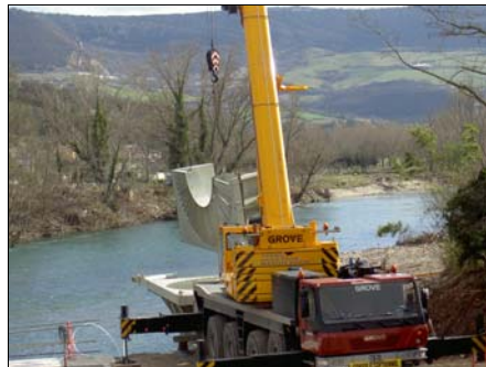
Assembly of the second distributor half
