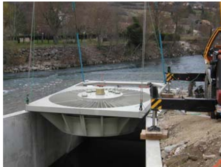
VLH in horizontal position above its final location
