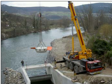
Transfer of the runner to the assembly area
