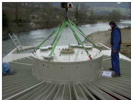
Assembly of the generator on the turbine shaft
