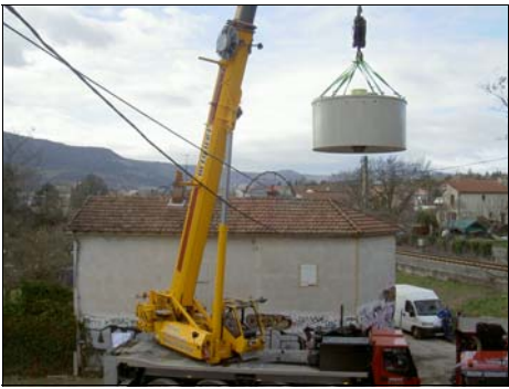
Unloading of the Generator
