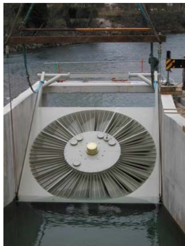
VLH in inclined position before opening gates
