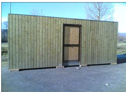
Huningue container equipment room
