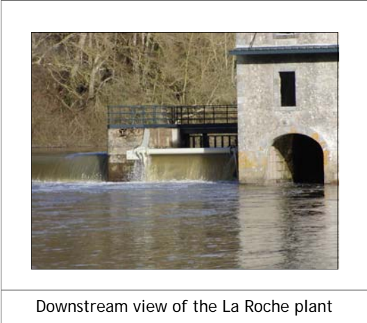
Downstream view of the La Roche plant with VLHs of the 14 other Mayenne locks and dams exploited by the SHEMA.
