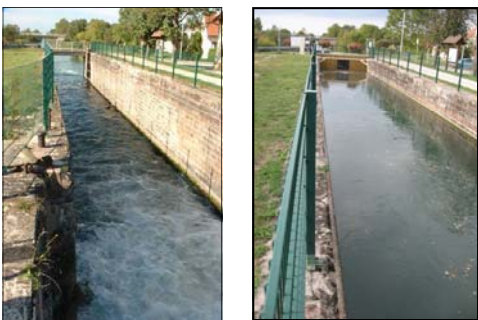
Before and after installation of the VLH
