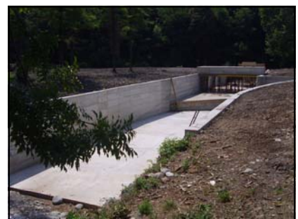
Water intake of the Vila d'Alme Plant
