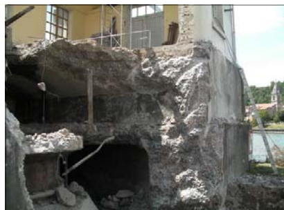
Demolitions downstream of the building
