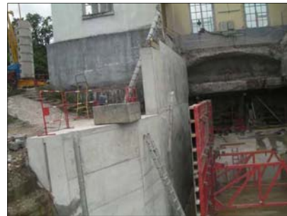
Building of the downstream right-hand side wall
