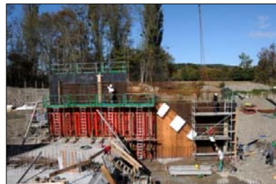
Les Barrets plant civil works
