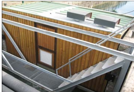
Rear view of the equipment room and of the access gangway
