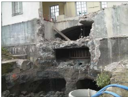
Demolitions downstream of the building
