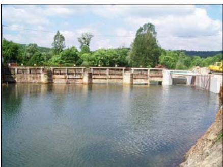
Clairvaux - upstream view of the water intake
