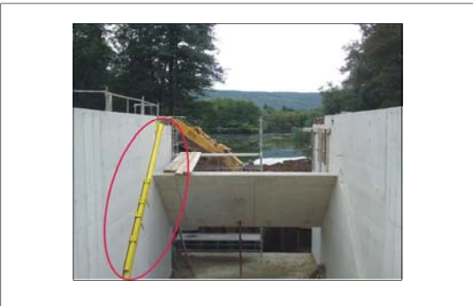
Placing of the parts to be sealed with the positioning tools provided by MJ2
