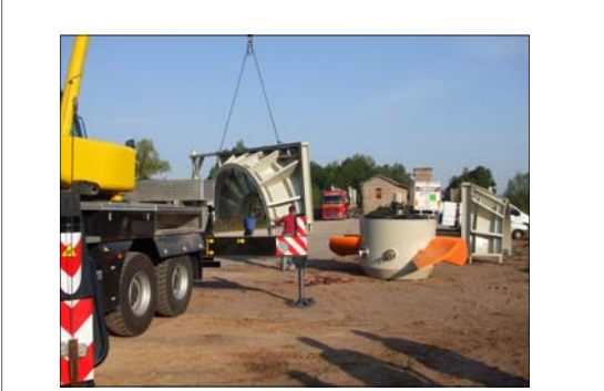
Unloading of a runner and of a half distributor
