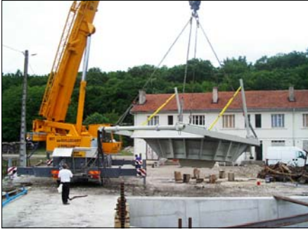
Installation of the VLH in its housing
