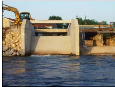
Downstream view of the Clairvaux power plant
