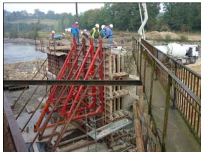
L'Ame plant civil works
